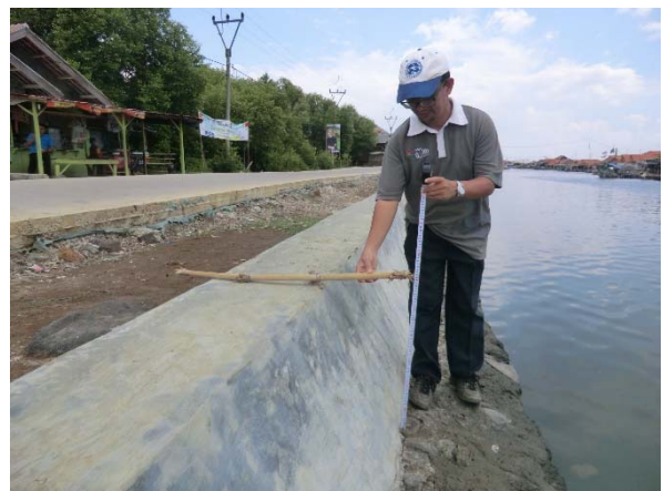
New seawall in Pondok Bali
